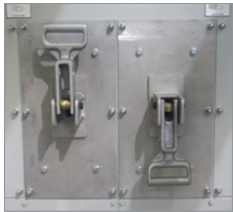
Furnace Selector Switches
