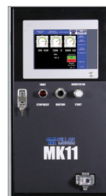
HMI Control Panel
