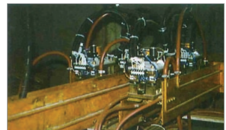
Furnace Selector Contactors
