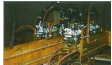
Furnace Selector Contactors
