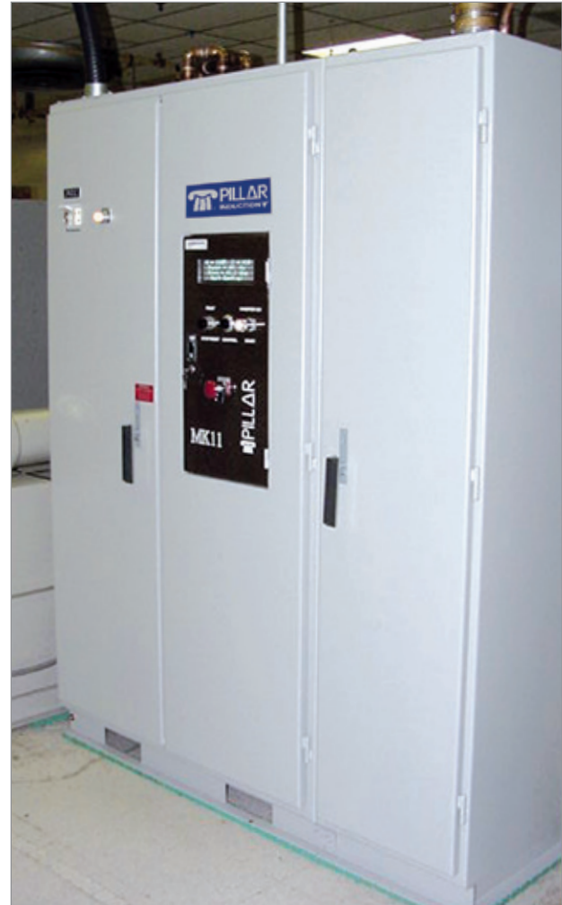
300kW – Size 2 cabinet (heat station attached)
